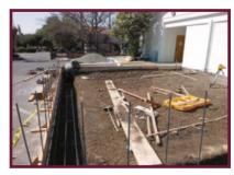
Paving has been removed from several parking spaces at the south end of the parish hall. A 5 to 6 foot high masonry wall covered with stucco and painted to match the church is being built to surround new air conditioning and heating equipment. When
