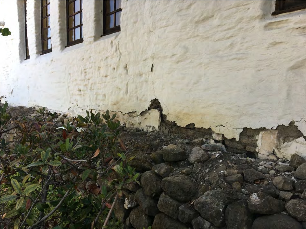
Detailed view of rock / adobe wall interface
