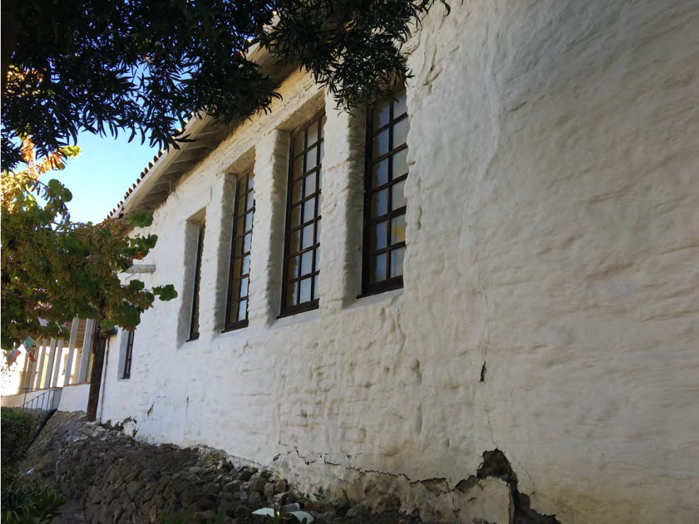
Closer view of West wall
